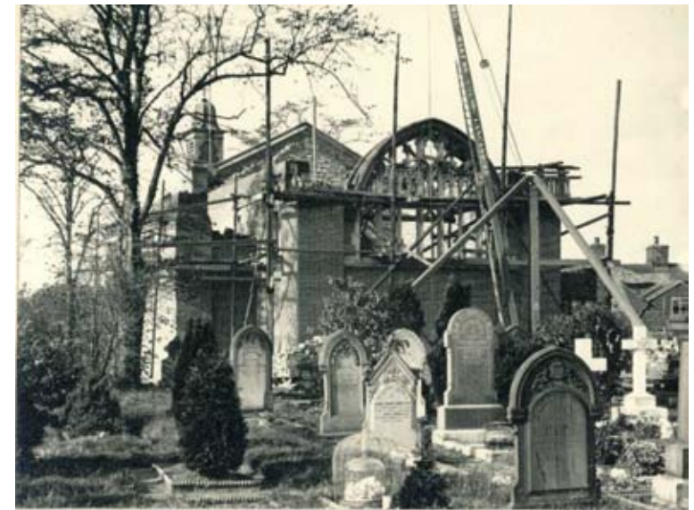
The building of the new chancel 1910
